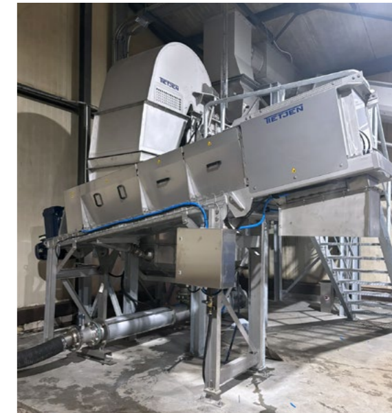
Installation of depackaging machine DRM and screw press PRS
